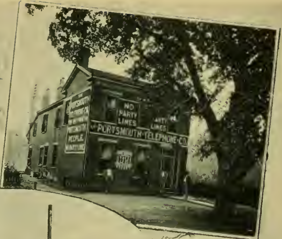
PORTSMOUTH TELEPHONE EXCHANGE
